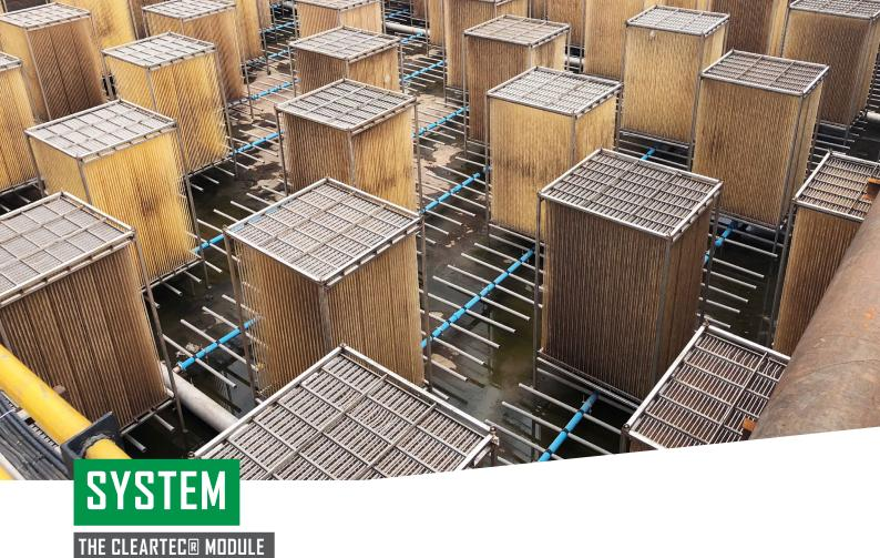
Cleartec® works as a system. The textile is fixed into a stainless steel cage, which can be assembled with aerators if required. A complete Cleartec® module consists of:
